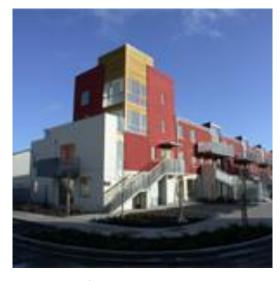
producing a lively elevational treatment, particularly in relation to the four-storey apartments. This Project clearly demonstrates the contribution a well developed precast concrete system can make to meeting this deman
