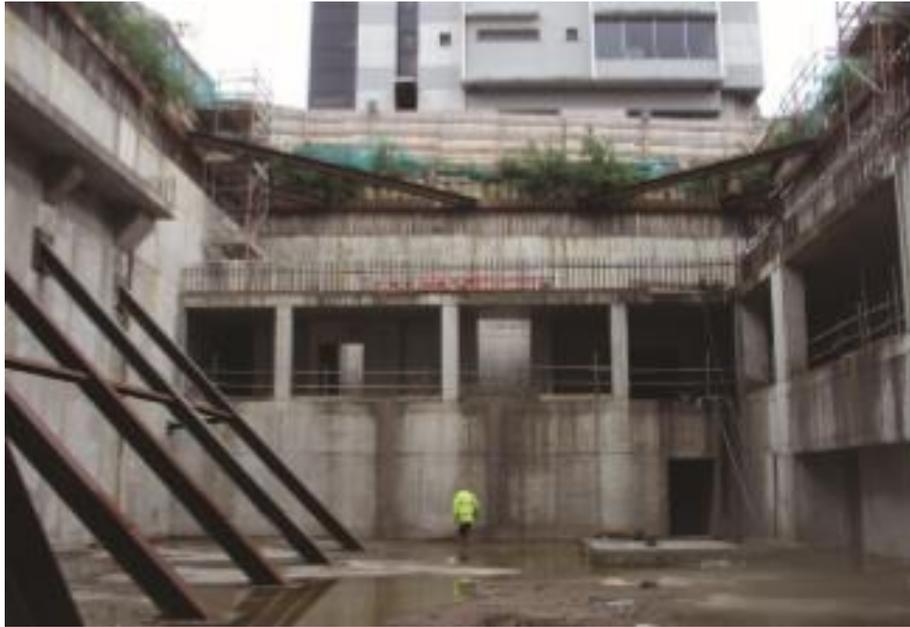
*Figure 4: Existing concrete box, with temporary support structures*
